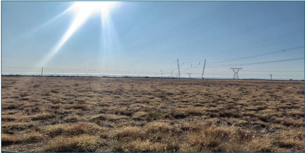
Figure 14: Areas surrounding the Ferrum substation
